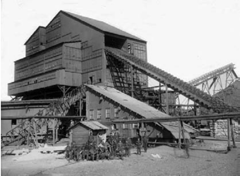
Figure 2.2. The “Iron Breaker” at Drifton No. 2, built by Eckley Coxe, circa 1891. To the upper right a conveyor deposits dirt and coal dust on a growing culm pile. Coal was hoisted from the mine along the ascending entrance to the top of the breaker, where it was washed, crushed to size, and picked clean by a workforce of “breaker boys,” some of whom posed here in front of the enormous building. Scanned from the negative by Eric Nystrom (2005), Division of Work and Industry, National Museum of American History, Smithsonian Institution.
