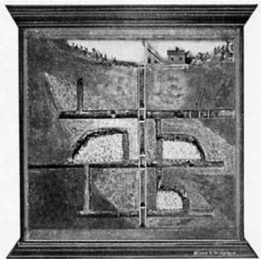
Figure 6.2. Walter R. Crane made this realistic model of a stope from concrete. He saw models like this one as important educational compromises between more-technical models that could not be understood without training, and inaccurate models that did not contain enough information to be instructional. From W[alter] R. Crane, "Concrete Mine Models," Mines and Minerals 27 (February 1907): 301.
